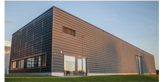
b.) Test Hall of the E.ON Energy Research Center in Aachen, Germany
